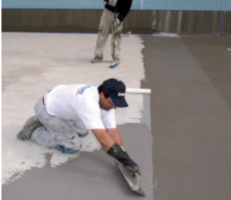
Hydroizolace bazénu Mapelasticem
